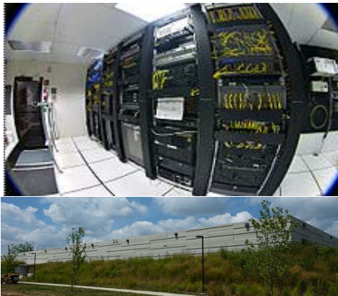
Indiana University Data Center. Bloomington, Indiana
